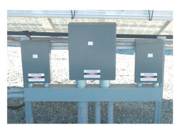
The optional StringWatch monitors solar PV system performance at the individual module, string, combiner box, and recombiner box levels, and automatically notifies the system administrator of any problems.
